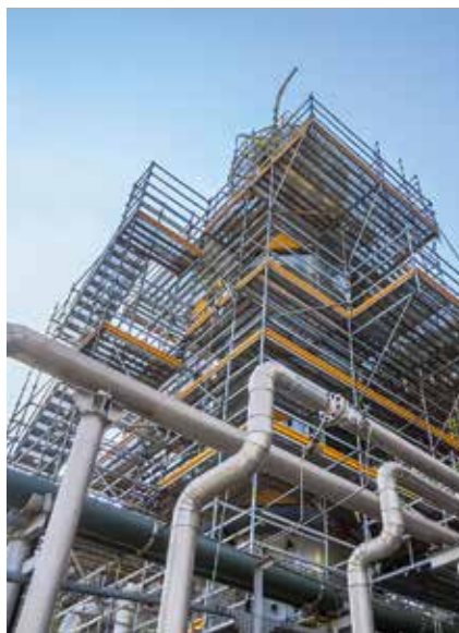
Stair towers with staircase units in the same direction have the advantage that, in addition to staircase units, working levels are also available.
